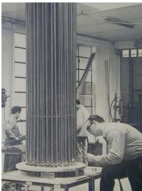
Braze Welding of the first flange-mounted heater Year 1967
